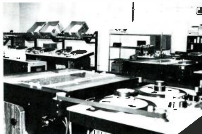
The Gauss loop bin and transport; this is one of five 1-inch, 1/2-inch, and Superscope-designed 1/4-inch loop bins in the facility.
